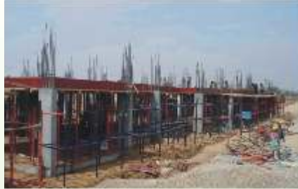
First floor slab framework at Plot 1,3,5&7 along Delonix street
