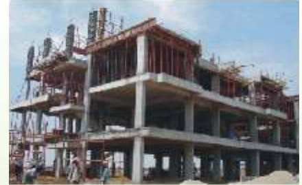
Columns upto roof slab casted at plots 18 & 20 along Delonix street
