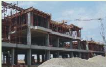
Third floor slab casted at plots 13&15 along Delonix street
