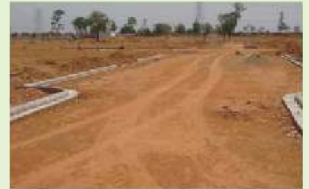
Street G, Lantana North Street
