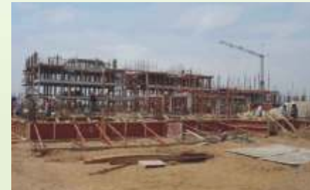
Plinth beams casting under progress at plots 19&21 along Ceiba street
